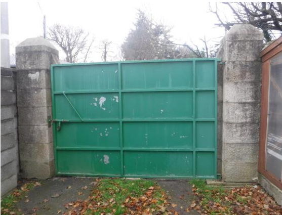
Photo 21: The vehicular gate as viewed from the east side
