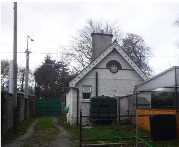
Photo 4: East gable of Woodbrook Side Lodge. The decorative timber bargeboards, brick dressings which have been painted over, and limestone plaque are original but the fenestration, cill and render are replacements
