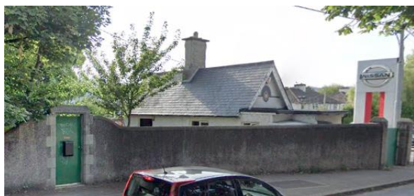
Photo 1: North and west elevations of Woodbrook Side Lodge as viewed from the Dublin Road
