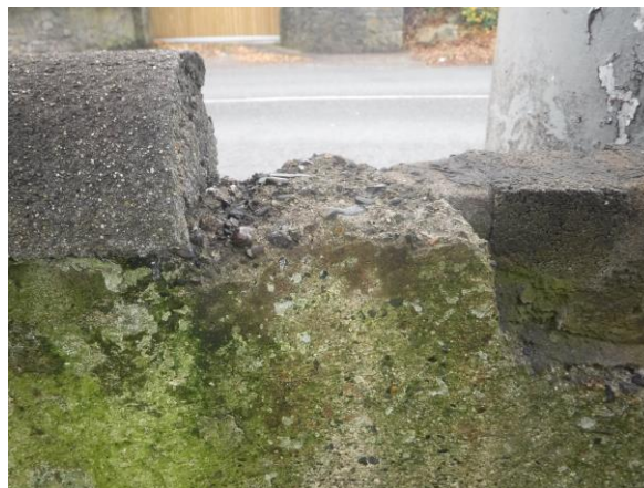
Photo 25 and 26: The east elevation of the boundary wall where the render and capping have fallen away, exposing the concrete block construction
