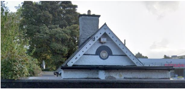
Photo 2: West gable of Woodbrook Side Lodge showing the, rendered and chamfered brick stack, decorative timber bargeboards, brick dressings which have been painted over, and limestone plaque
