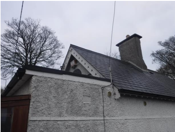
Photo 8: The flat roofed extension to the west gable of Woodbrook Side Lodge. The extension is a 20th century addition of no heritage value and obscures the west gable and barge boards
