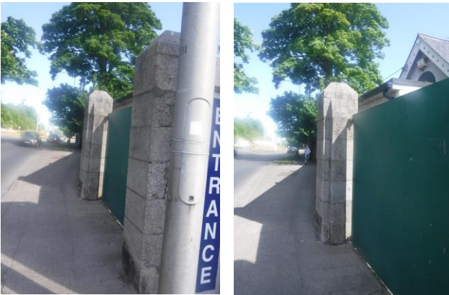
Photo 19 and 20: The vehicular gate as viewed from the west or Dublin Road side
