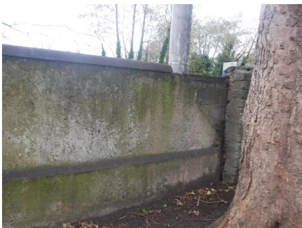
Photo 25 and 26: The east elevation of the boundary wall where the render and capping have fallen away, exposing the concrete block construction
